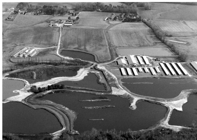
Confined animal feeding operations in eastern North Carolina showing fecal waste pits (foreground), confinement structures (left and right middle), spray fields, and neighboring homes
